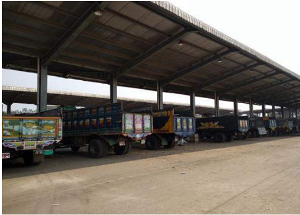
Pic 5: Transshipment Shed Facilities
