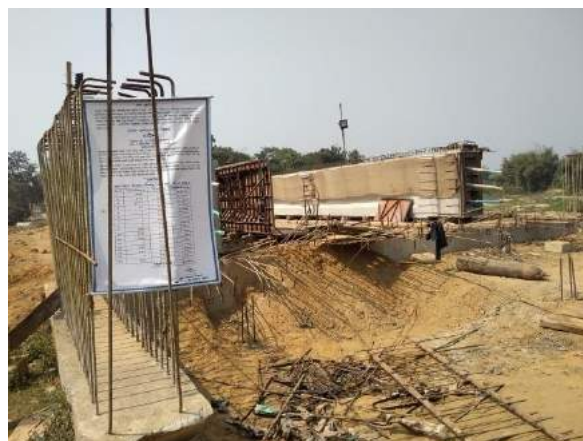
Pic 44: Road Improvement Activities
