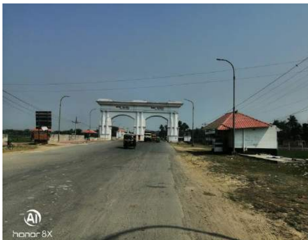
Pic 19: Access Roads Border on Bangladesh Side
