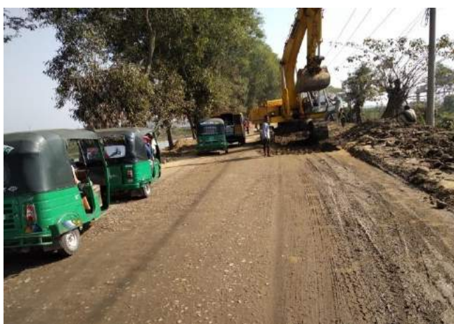
Pic 41: Road Improvement Activities
