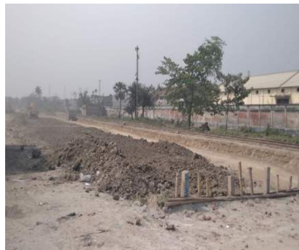
Pic 20: Road Extension Activities at Benapole Land Port
